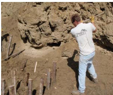
Phil Carter pounds pickets to create one of several wood baffles completed.
