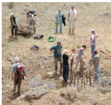
On the scene of baffle construction.
