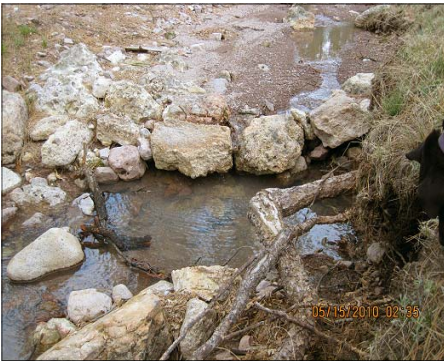
Here's one of our previous one-rock dams operating just as designed: sediment has accumulated upstream of the structure, slowing water flow and raising the channel level.
