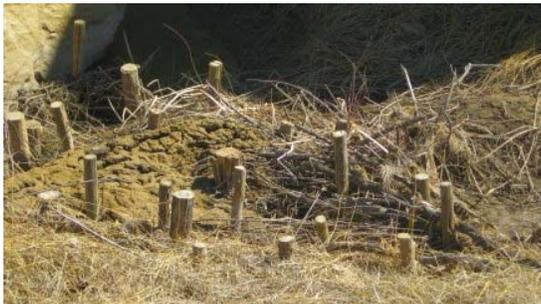
One of last year's wicker baffles doing its job— capturing debris and sediment and shifting the course of the creek toward the arroyo wall.
