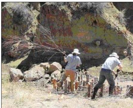
Branches are woven into the baffle to trap sediment.
