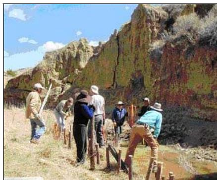
About 45 pickets are pounded into the channel to form a baffle.
