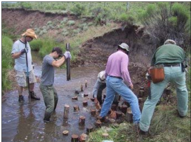
BUILDING A POST VANE: Left to right, Bob Tilley rests after drilling a starter hole with a rock bar, as Chris Sanderson pounds down another post. Bill Zeedyk crouches to place a stabilizing stone between posts, while Gene Tatum and George Long pass along additional rocks.
